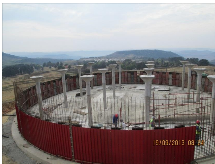
Figure 4-3: Concrete Reservoir under Construction
