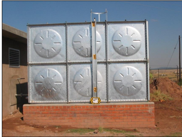
Figure 4-1: Typical Pressed Steel Tank as Reservoir
